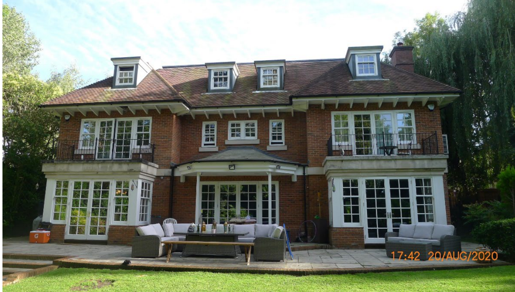
Figure 2: Rear elevation of the existing house
